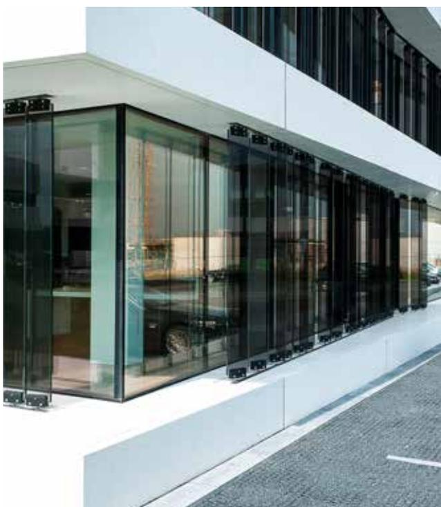
Eyecatcher here is the minimalistic window Artline which is used almost throughout the whole building, allowing natural light to illuminate the offices inside.
